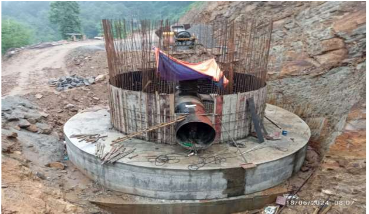
Figure 9: Surge tank foundation.
