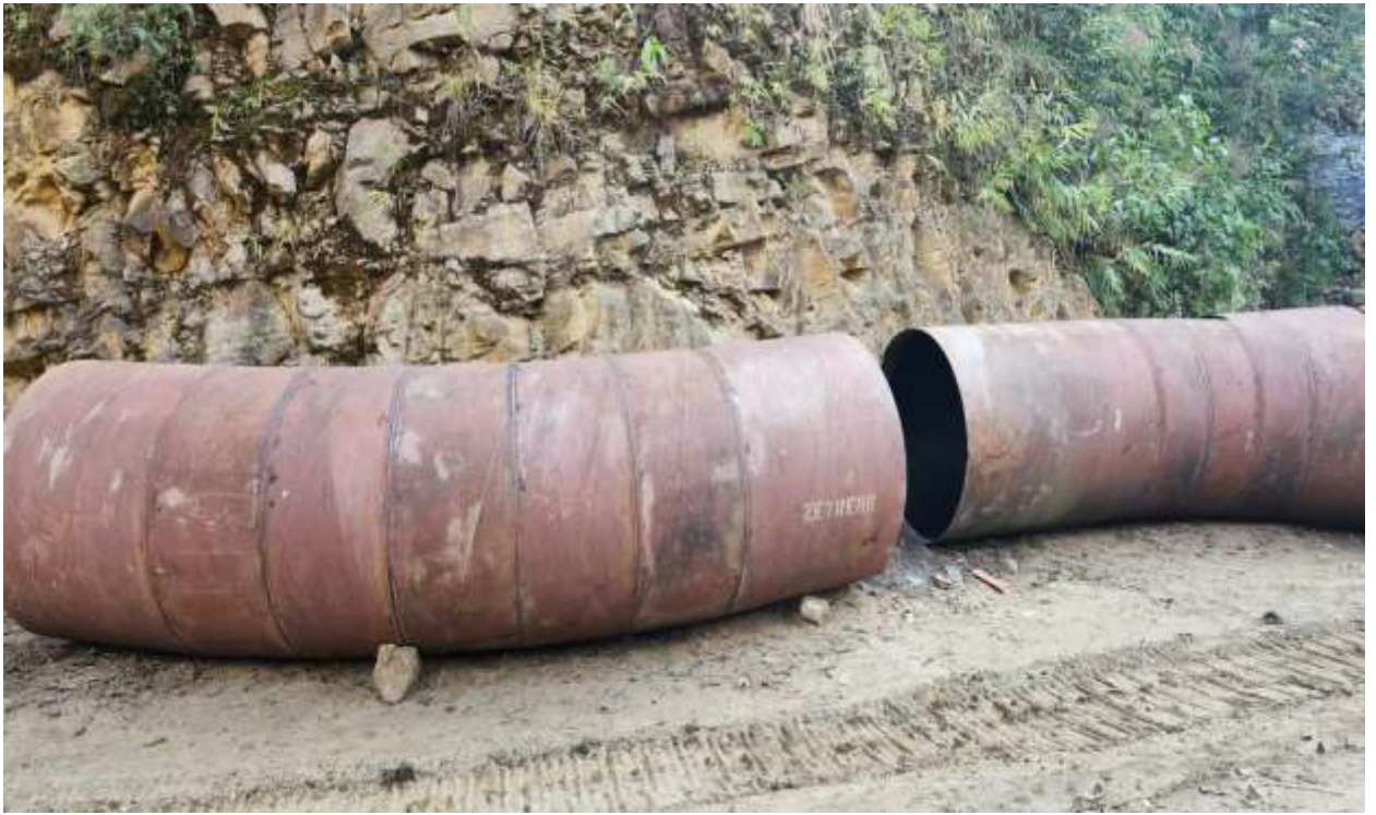
Figure 17: Bend ready for remaining Headrace alignment.
