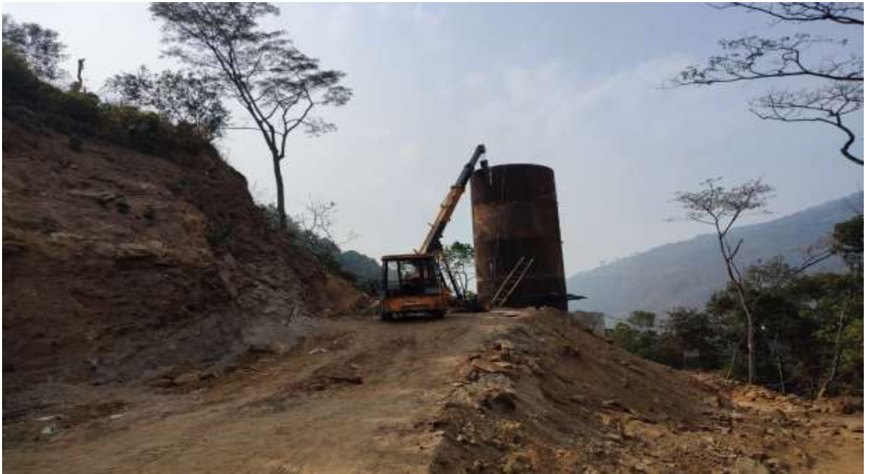
Figure 21: Installation pipe sections for surge tank.
