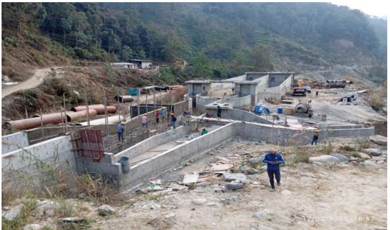
Figure 4: Gravel Settling basin after completion.
