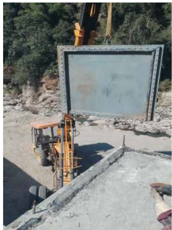
Figure 25: Gate and hoisting installation work.
