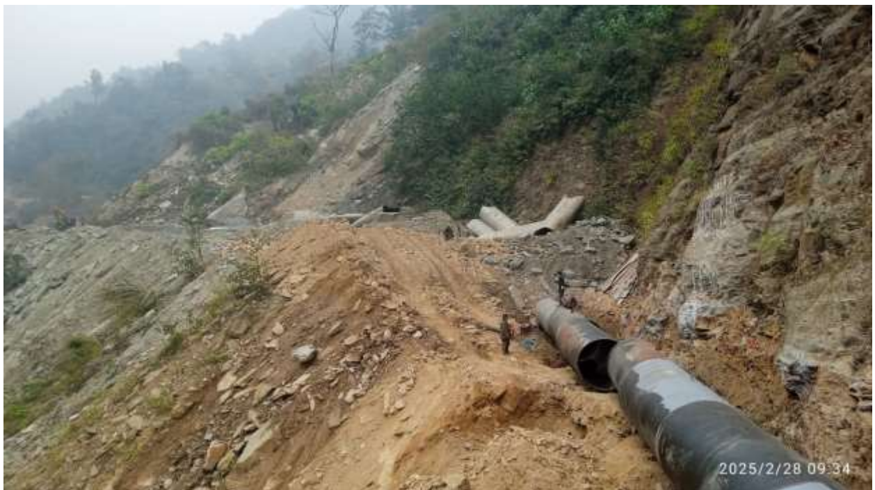
Figure 7: Syphon after final protection.
