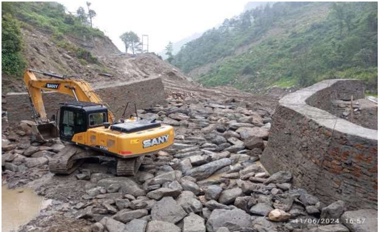
Figure 7: Syphon after final protection.
