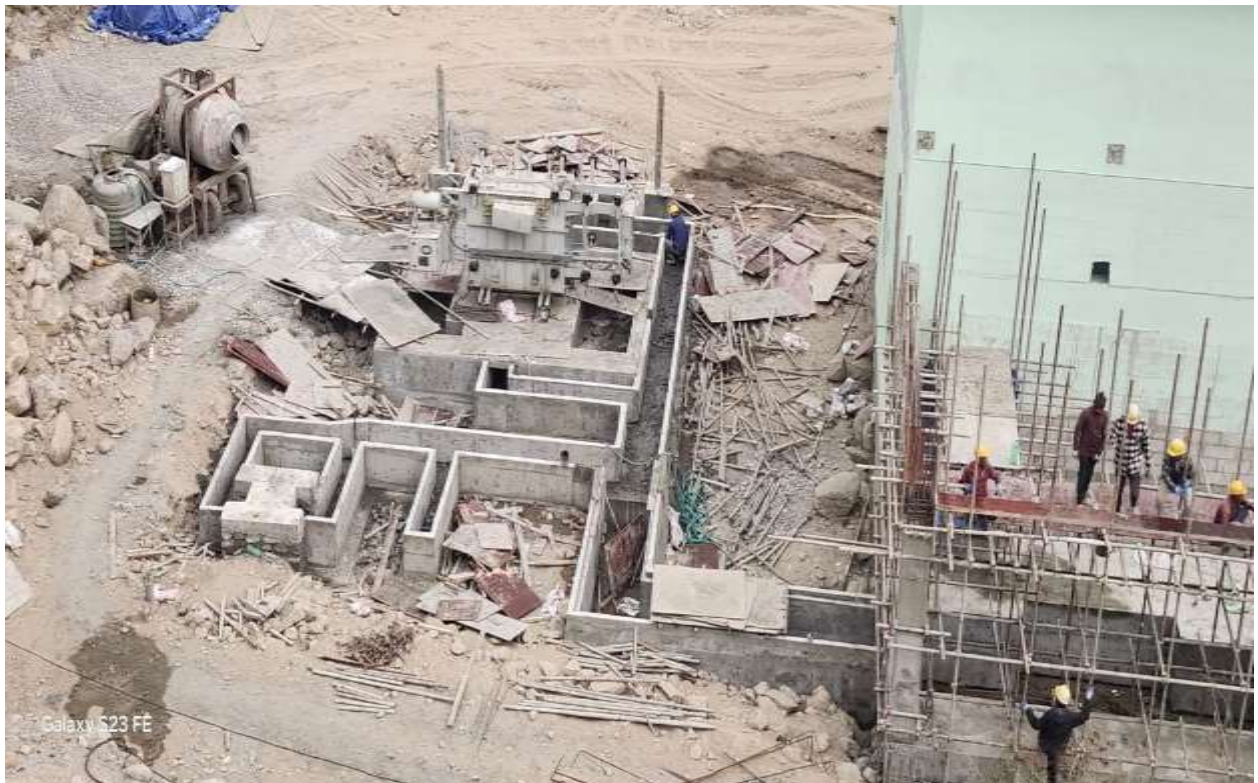
Figure 12: Transformer foundation and switchyard area after completion.
