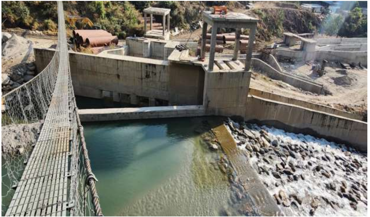
Figure 3: Intake and undersluice.
