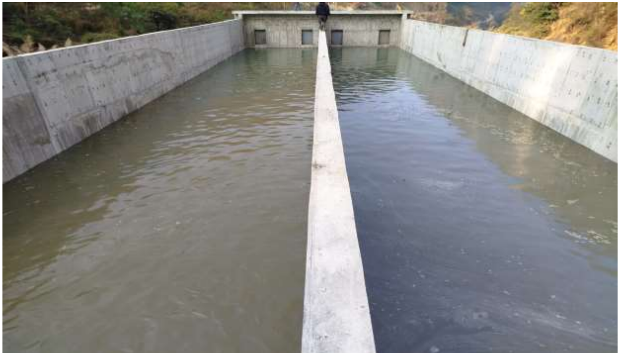
Figure 5: Forebay structure after completion.
