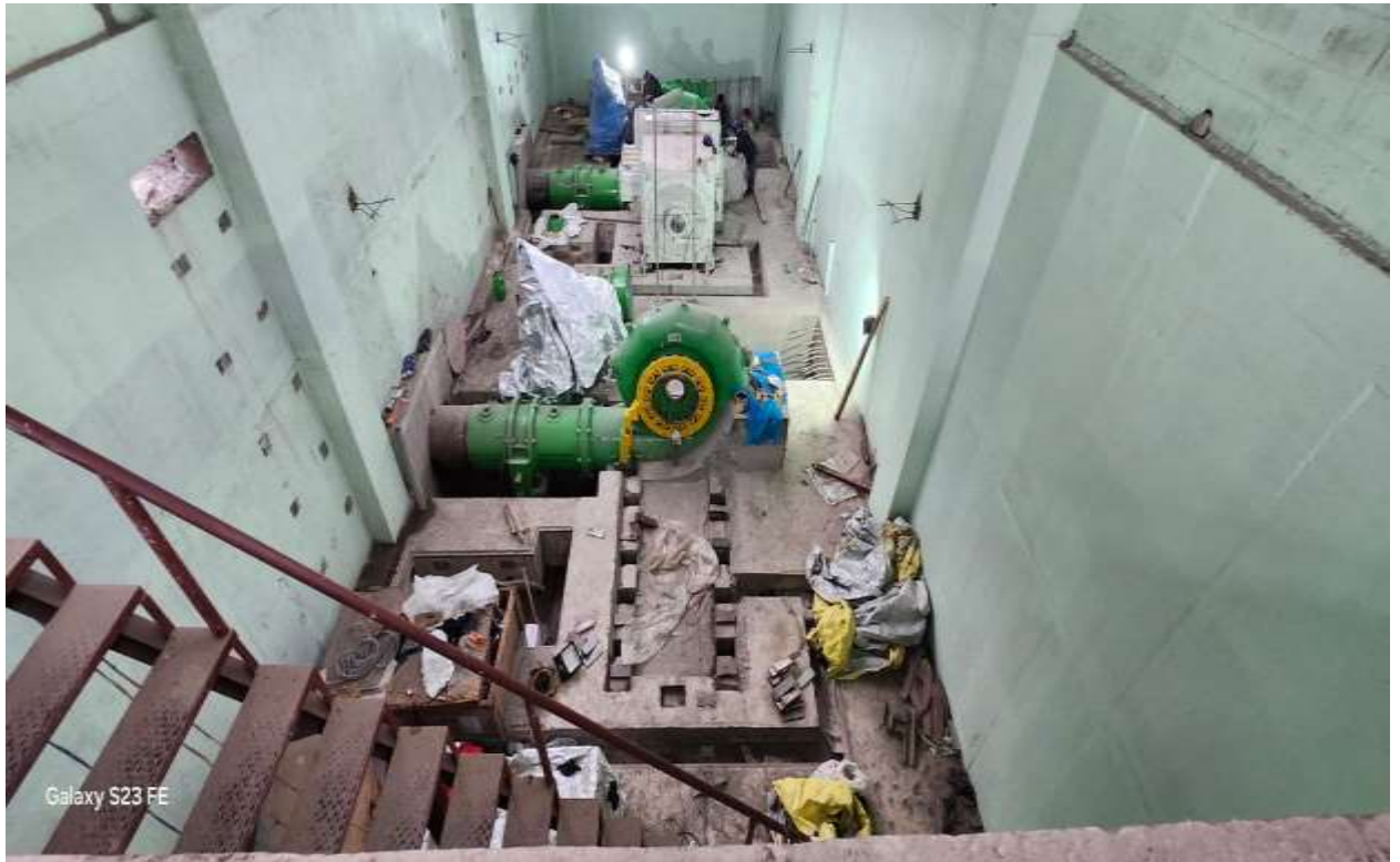
Figure 13 : Machine Installation work.
