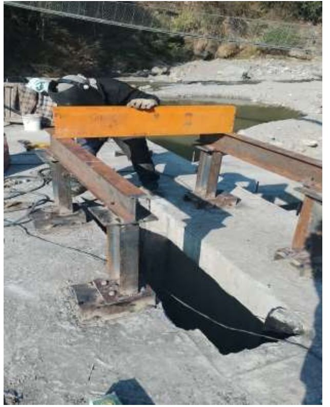
Figure 25: Gate and hoisting installation work.
