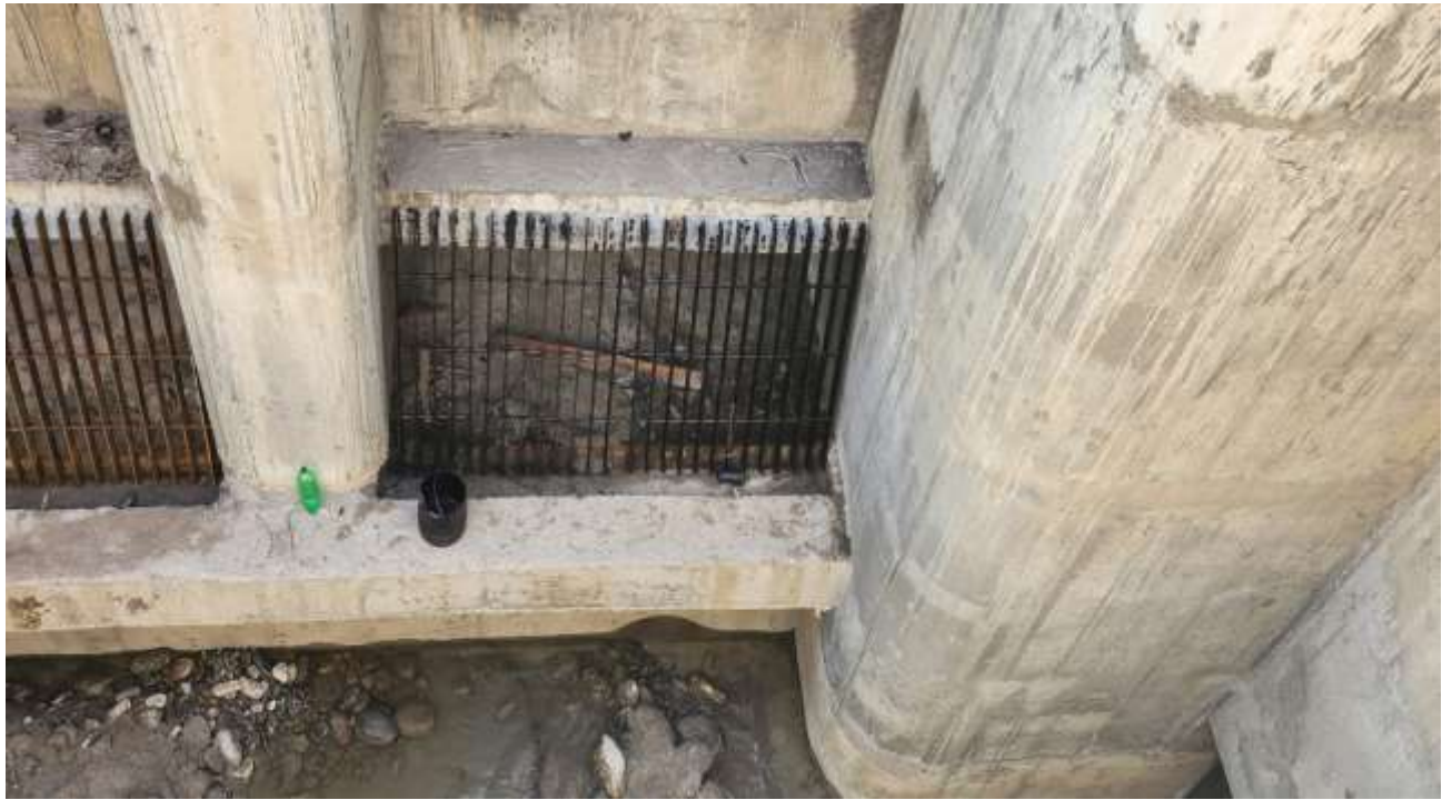
Figure 28: Trash rack installation at intake.
