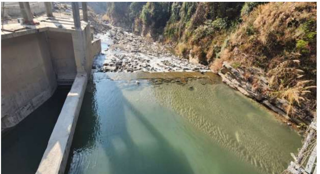
Figure 27: Water Filling after gate installation.
