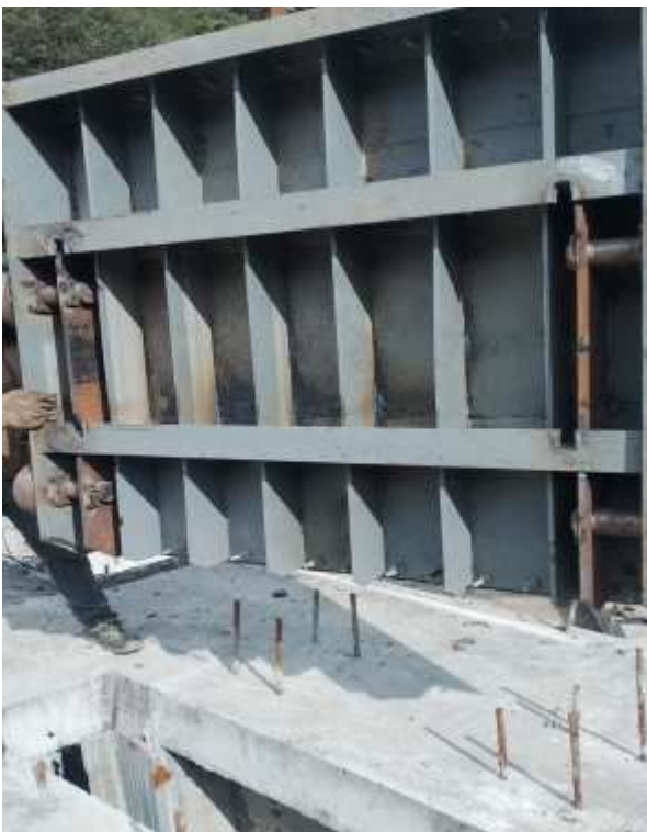
Figure 25: Gate and hoisting installation work.
