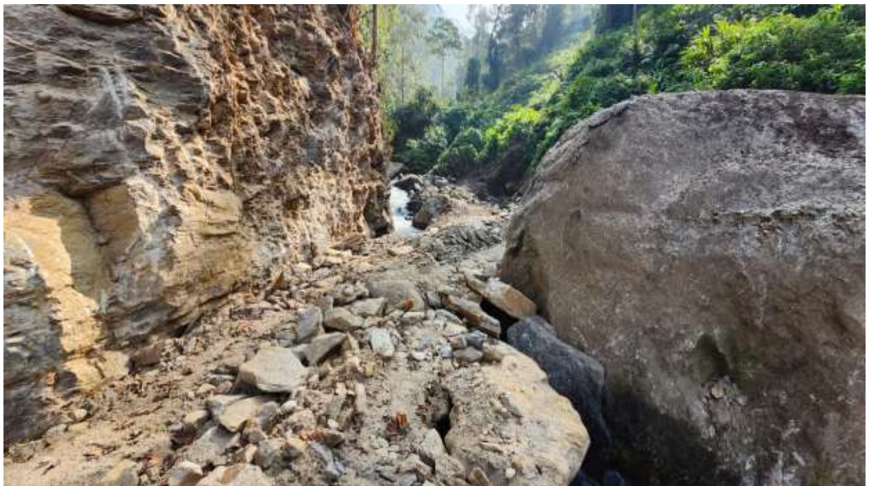
Figure 16: Excavation for Sikhuwa Diversion
