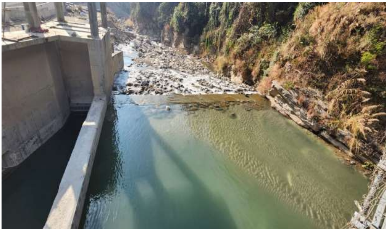
Figure 2: Weir and undersluice downstream side.
