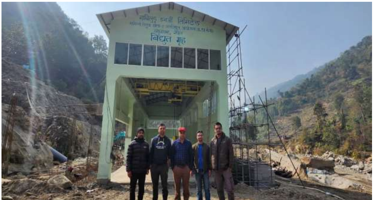
Figure 33: Site visit of technical consultant along with client team.
