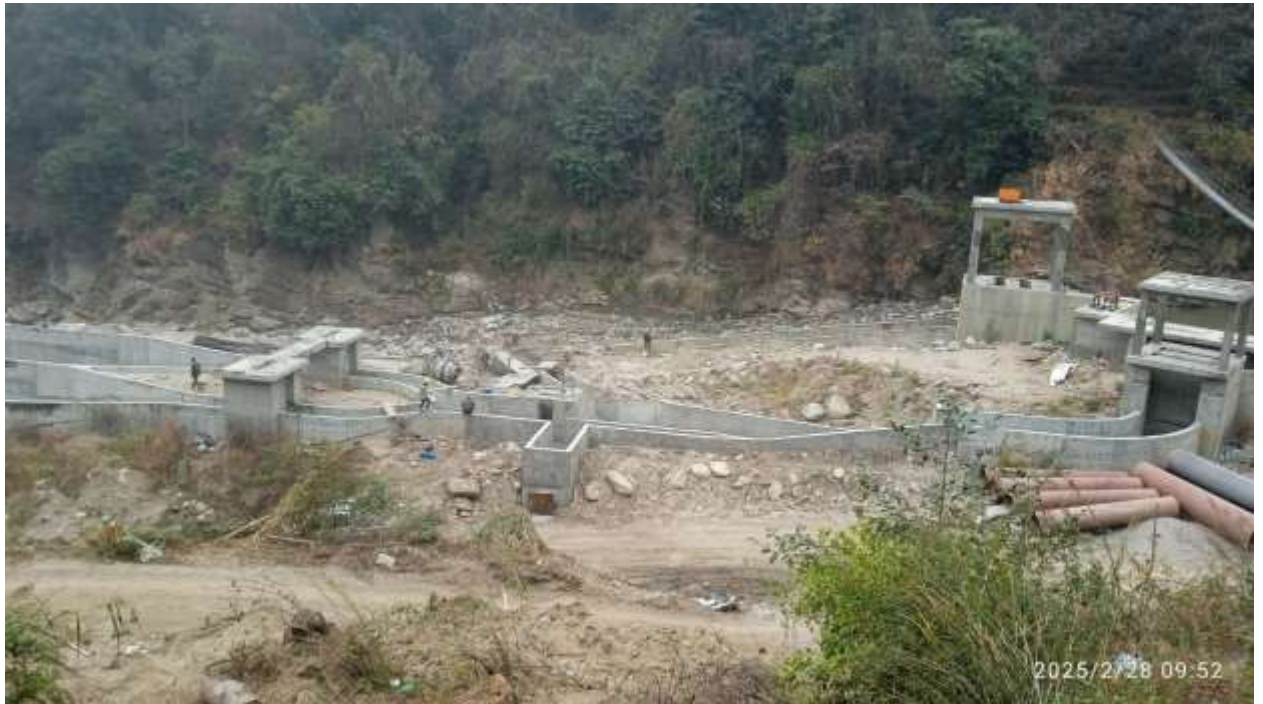
Figure 5: Forebay structure after completion.
