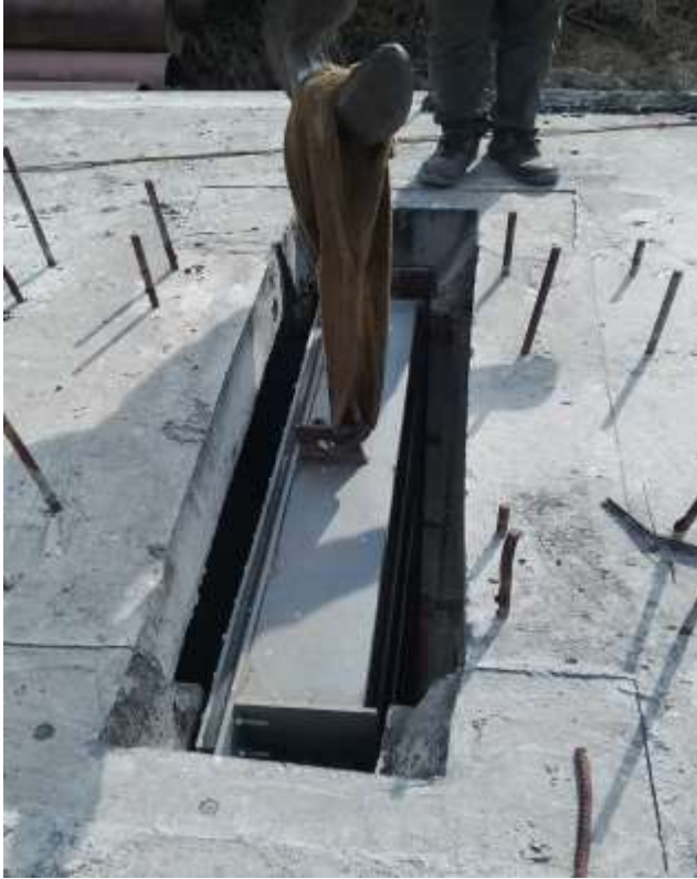
Figure 25: Gate and hoisting installation work.
