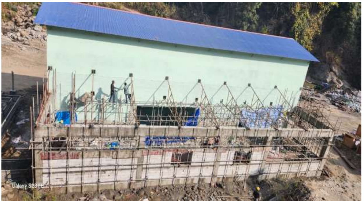
Figure 14: Control room in final stage of construction.
