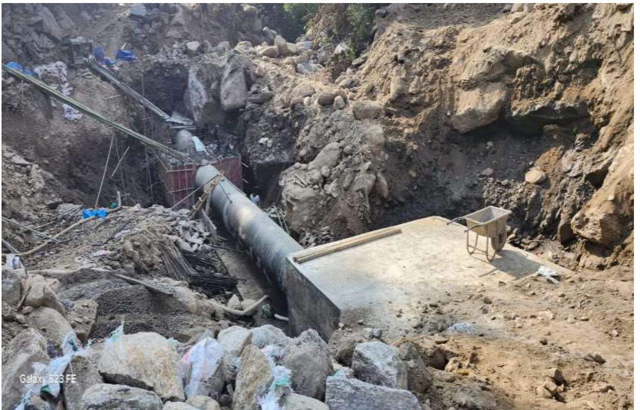
Figure 20: Lakuwa Crossing near powerhouse.
