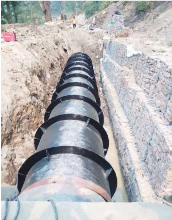
Figure 19: Pipe Installation and protection work.
