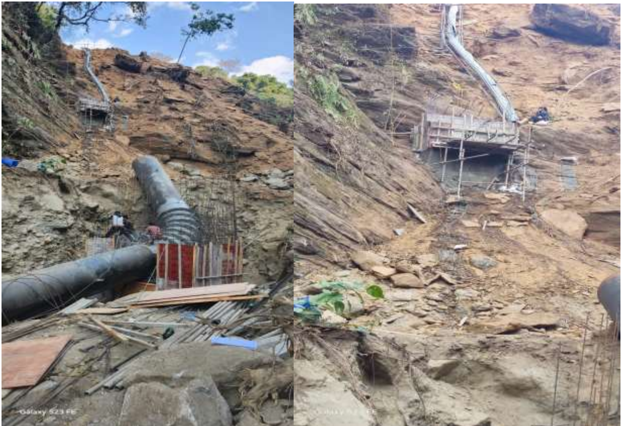
Figure 22: Installation bend , saddle support and penstock pipe at vertical section.
