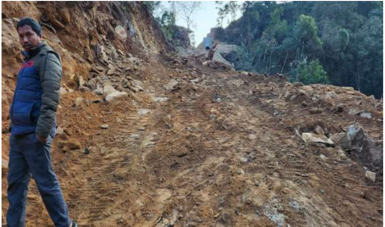
Figure 15: Excavation of Penstock Alignment.
