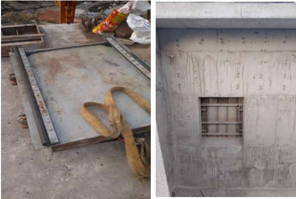
Figure 26: Gate installation work.
