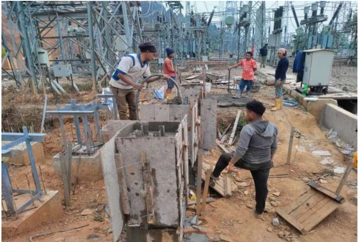
Figure 32: Substation foundation and superstructure installation work.
