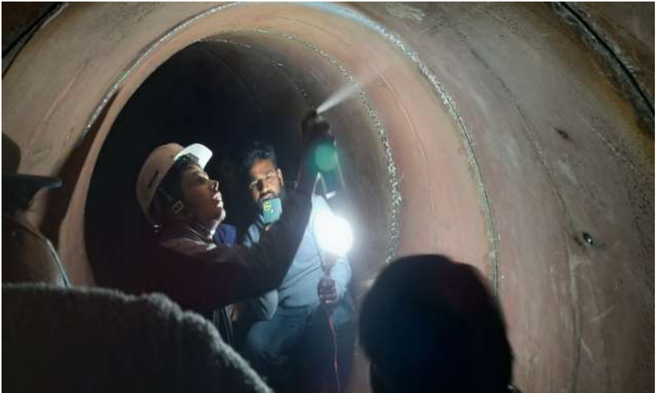
Figure 23: NDT test in pipe welding.
