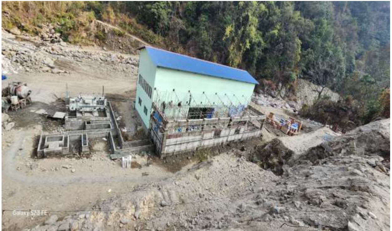
Figure 11: Overall Powerhouse area.
