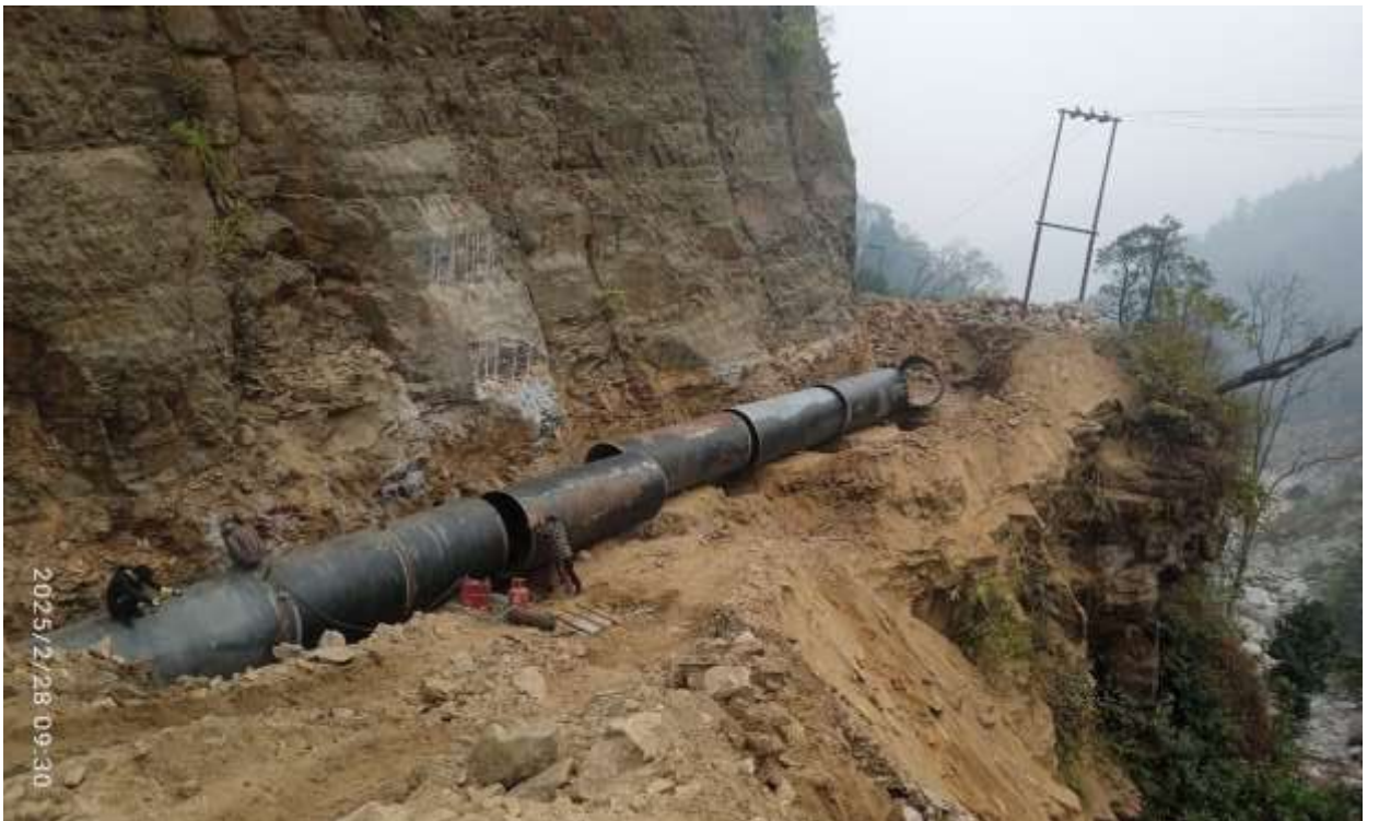
Figure 18: Headrace pipe installation around landslide Rocky area.
