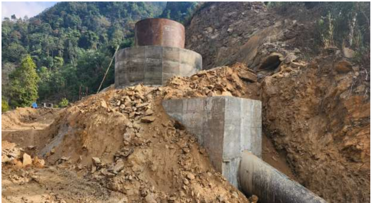
Figure 10: Surge tank civil works on final stage of completing.
